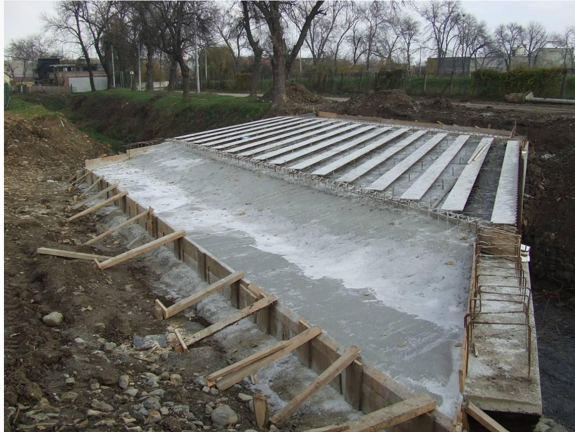
Foto 4. Partially concreted carriage way and transition plate
